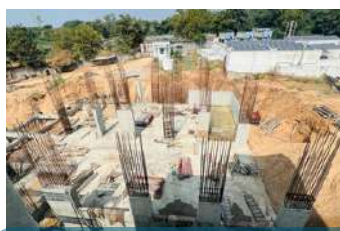
Construction of CoEN Building
